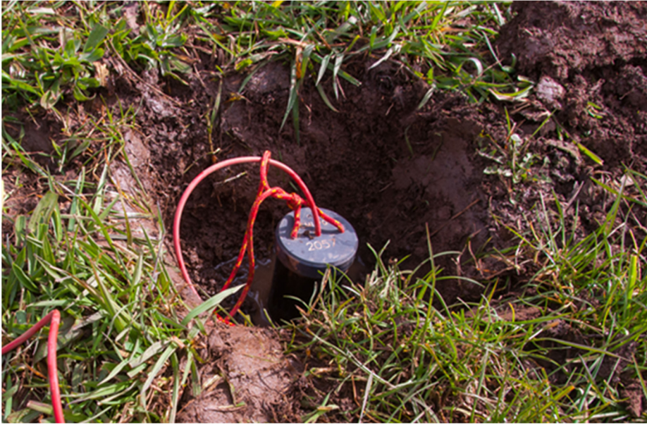
Figure 5: LEMI-701 Cu/CuSO 4 electrode installed in a hole (before burying, shown at shallower depth for visibility).
